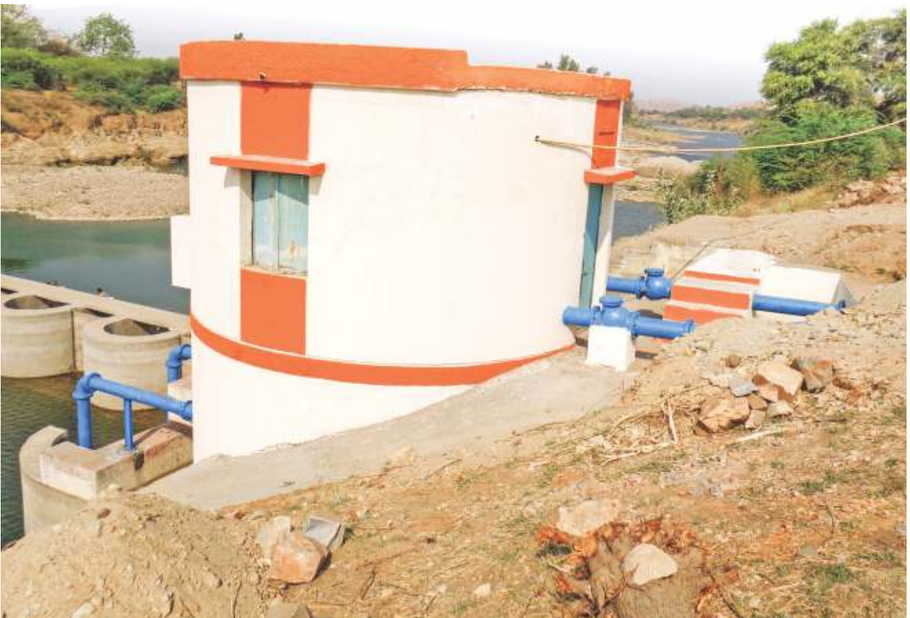
Repaired Pump house and delivery pipe of Vanjharia Lift Irrigation Scheme, Dahod
