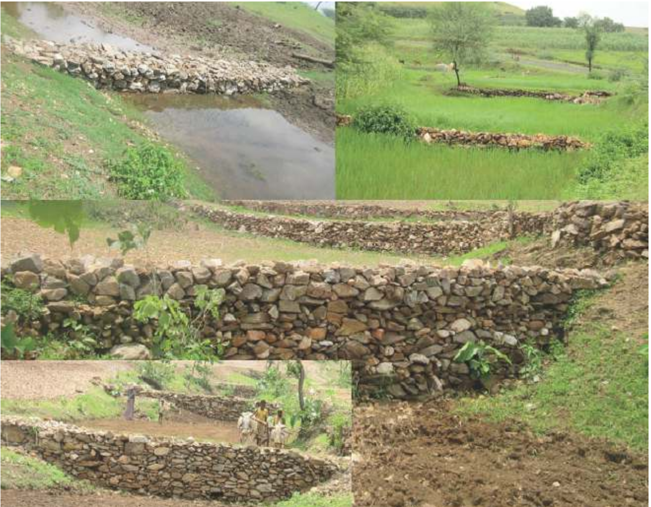
Drainage Line Treatment in Watershed in village Jhalakiya, Banswara, Rajasthan
